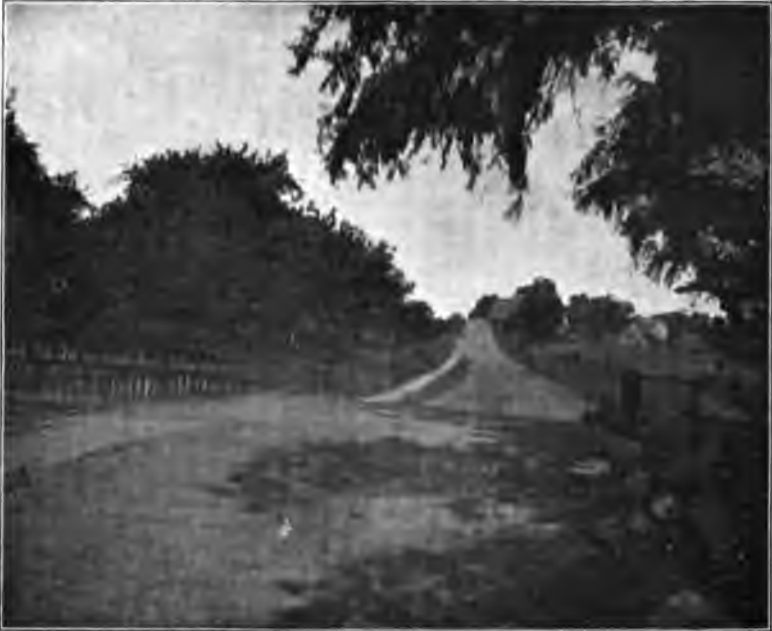
Stewartville road, Warren Co., before improvement.
